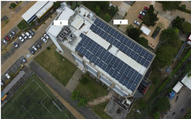
Fig. 2. Rooftop solar photovoltaic installation for the case study.
