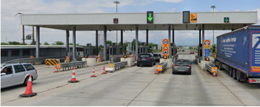
Fig. 3. Iasmos toll station, direction from Igoumenitsa to Kipi/Alexandroupoli.
